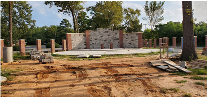
Altar Area: cleared to install a new granite Altar
