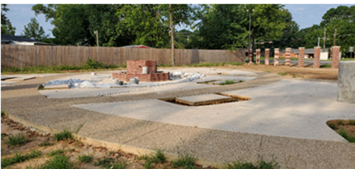
The Center of Columbarium - being built for Pietà Statue with a fountain installed for ever-flowing 'Water of Grace.'
